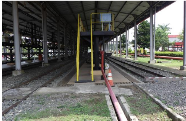
Fig. 1. Area Filling Shed Rail Tank Wagon Fuel Terminal Rewulu
