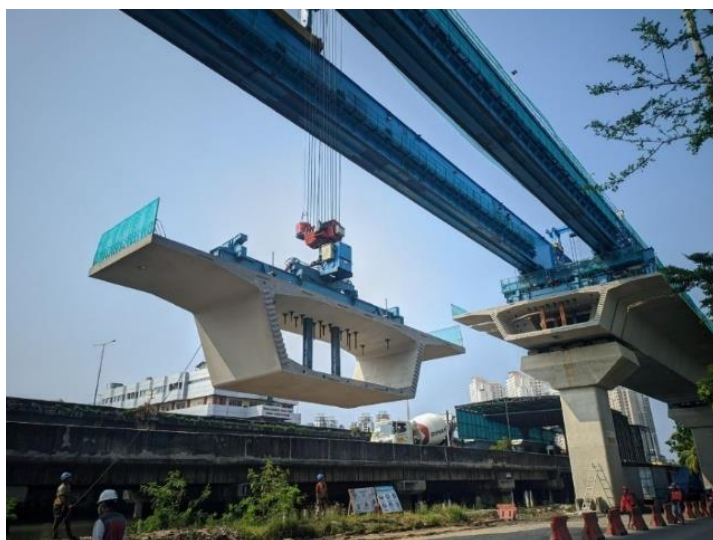
Figure 2. Erection box girder
