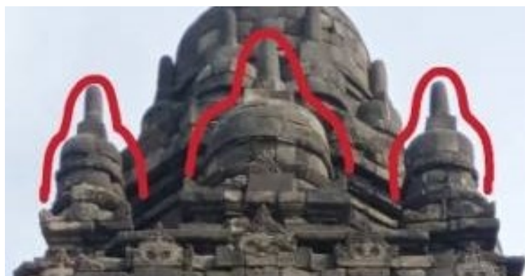
Figure 2.2. The roof of Sewu Temple
