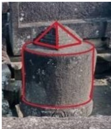
Figure 1.1. The roof of the Sewu Temple
