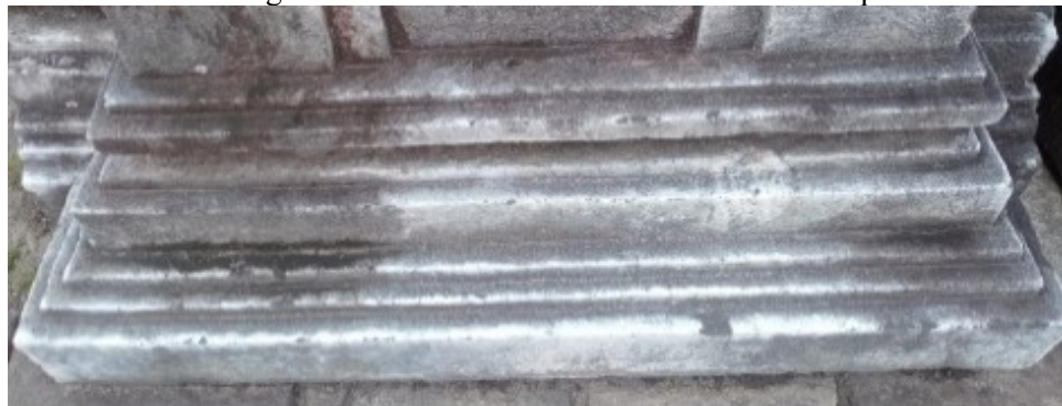
Figure 3.2. The Upper Wall of Sewu Temple
