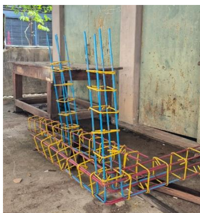
Figure 3. Column and Tie-Beam Reinforcement Assembly
