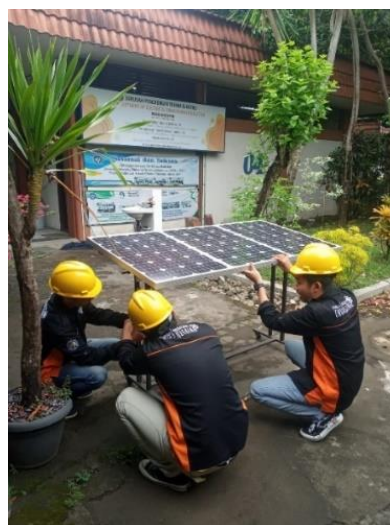
Fig. 6. Solar panel assembly
