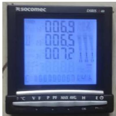
**Fig. 1.** Voltage THD on incoming 6KV panel
