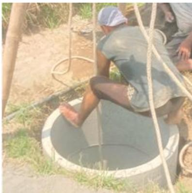
**Figure 10.** Precast concrete ring installation
