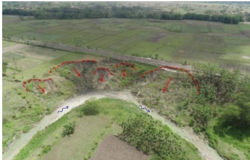
Figure 2. Landslides in the study area.
