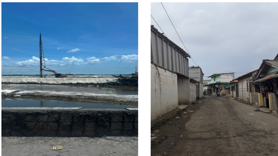
Figure 1. Sand Dredging & Conditions of Village
