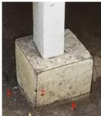
Figure 8. The foundation of Kampung Pulo traditional house
