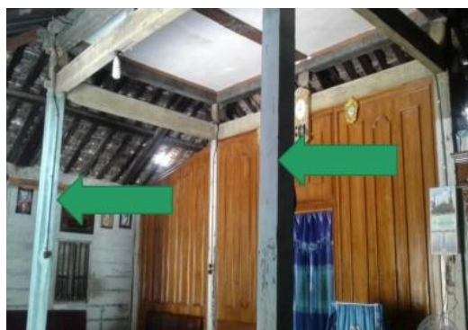
Figure 11. The main pillar of the Joglo traditional house in Sumurpule Village, Pati
