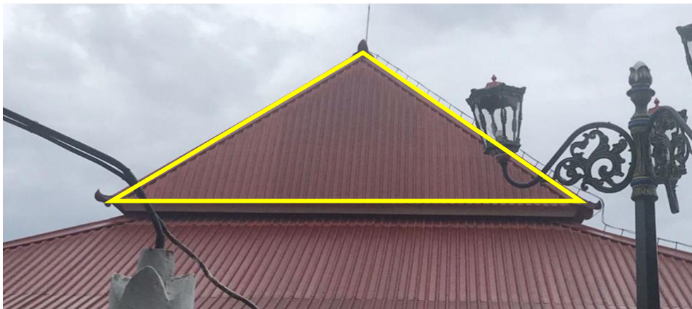
Figure 3. A triangle (on the roof)
