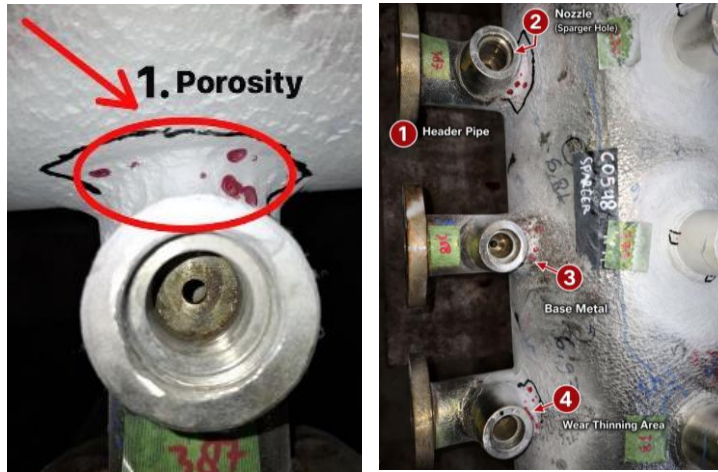
Figure 2. LPT results showing surface indications on the weld area
