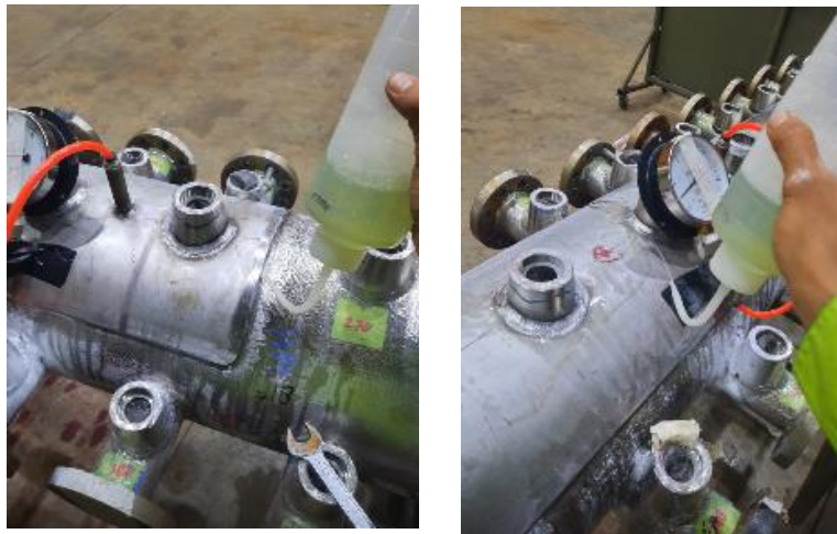
Figure 5. Leak testing setup/result of sparger header RE-C215
