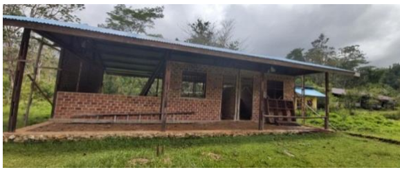
Picture 1 : church house of worship construction.
