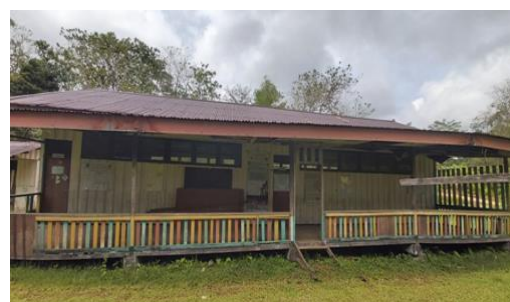
Picture 3 : School renovation
