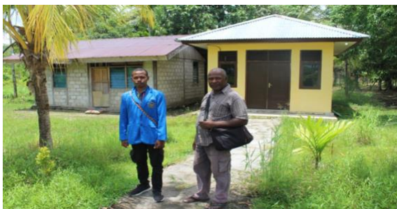
Picture 6 : construction of an old house into a new house.
