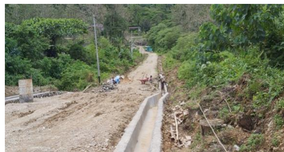
Picture 5 : Irrigation and road construction.
