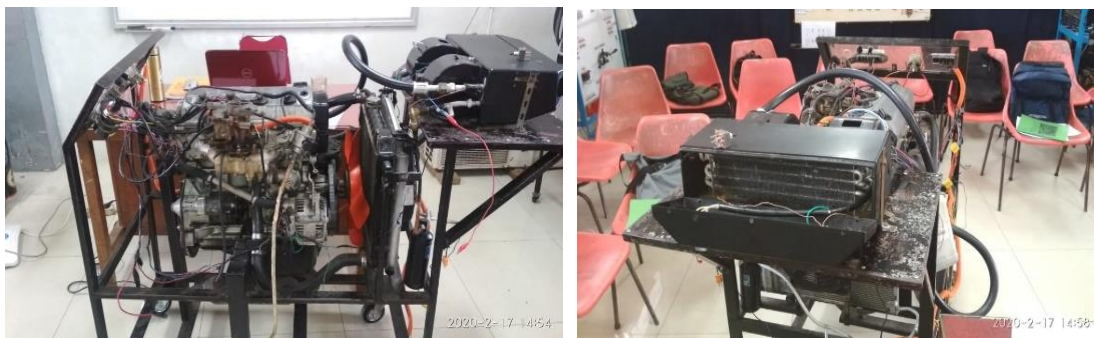
Figure 1. The condition of the air conditioner (AC) practicum equipment which was heavily damaged and produced pollution during practical activities
