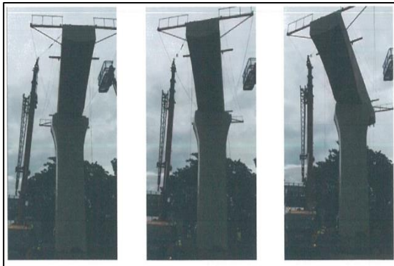
Fig. 7. The momentum of Erection for Pier Head structure
