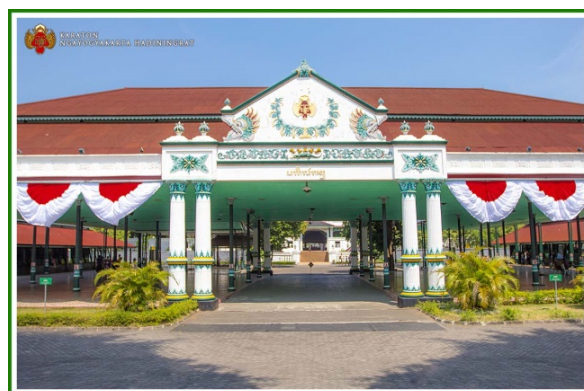
Figure 1. The Facade of the Palace has a Distinct Traditional Yogyakarta Shape Serves as a Learning Resource for Combination of Two-Dimensional Shapes and Three-Dimensional Figures (Measuring)
