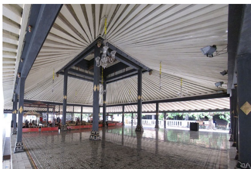
Figure 5. The Design of the Bangsal Manganti Hall with Traditional Javanese Architecture Serves as a Mathematics Learning Resource for Lesson of Area and Perimeter (Measuring)
