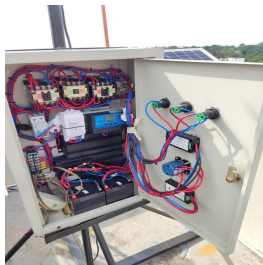
Figure 6. WPP, SPP, PLN panel network
